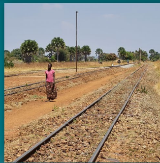
New railway line between Dar es Salaam and Mwanza. Section: Tabora – Isaka Tanzania
