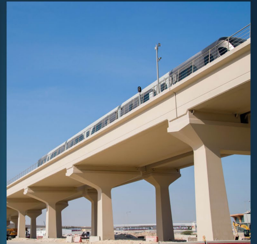
▲ Doha Metro Network, Qatar
