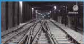
Double crossover installed in Metro Buenos Aires
