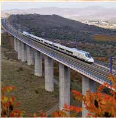
Spanish High Speed Network. Design & Construction Supervision Services
